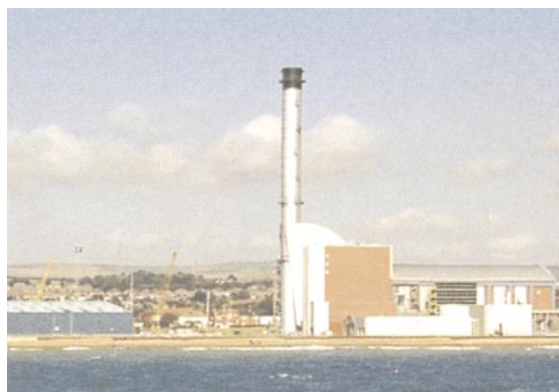
Shoreham Power Station
