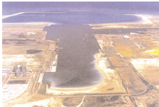
Dunkerque—Port Ouest from S
