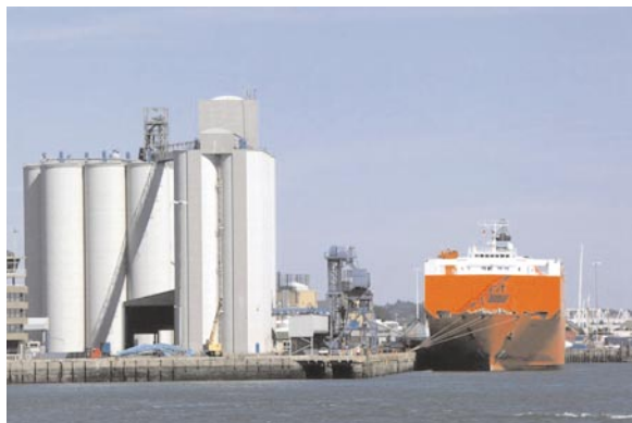
Eastern Docks Silo
