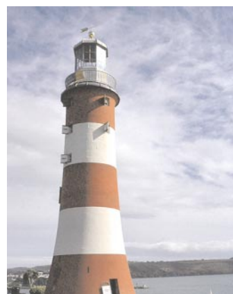
Smeaton Tower (disused)
