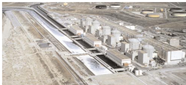
Gravelines Nuclear Power Station
