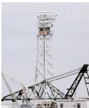
Admiralty Jetty Radar Tower
