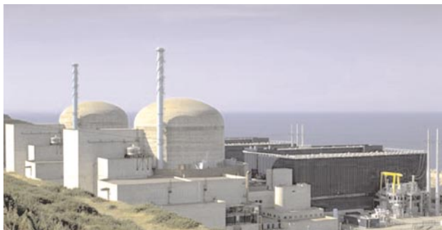
Flamanville Nuclear Power Station
