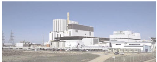
Dungeness Nuclear Power Station
