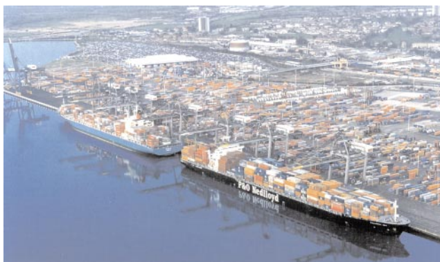
Southampton Container Terminal
