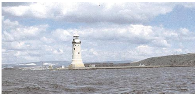
Plymouth Breakwater West Light
