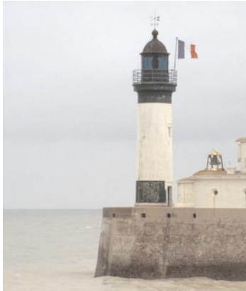
Le Treport Light (West Breakwater)
